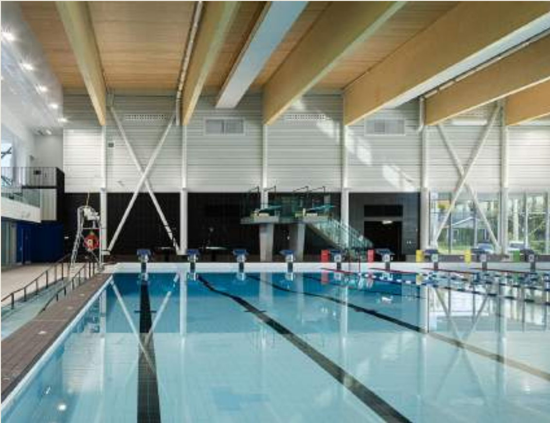
St-Georges multisports complex, QC by Structure Fusion
