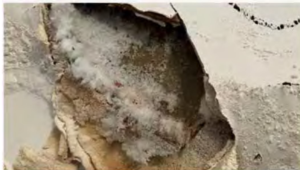
This home in County Durham had external wall insulation fitted in 2021
