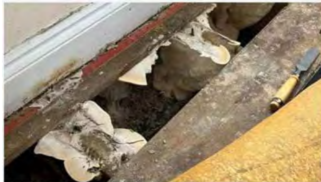
A family in Luton has been forced to move out as dry rot fungus grows under the floor
