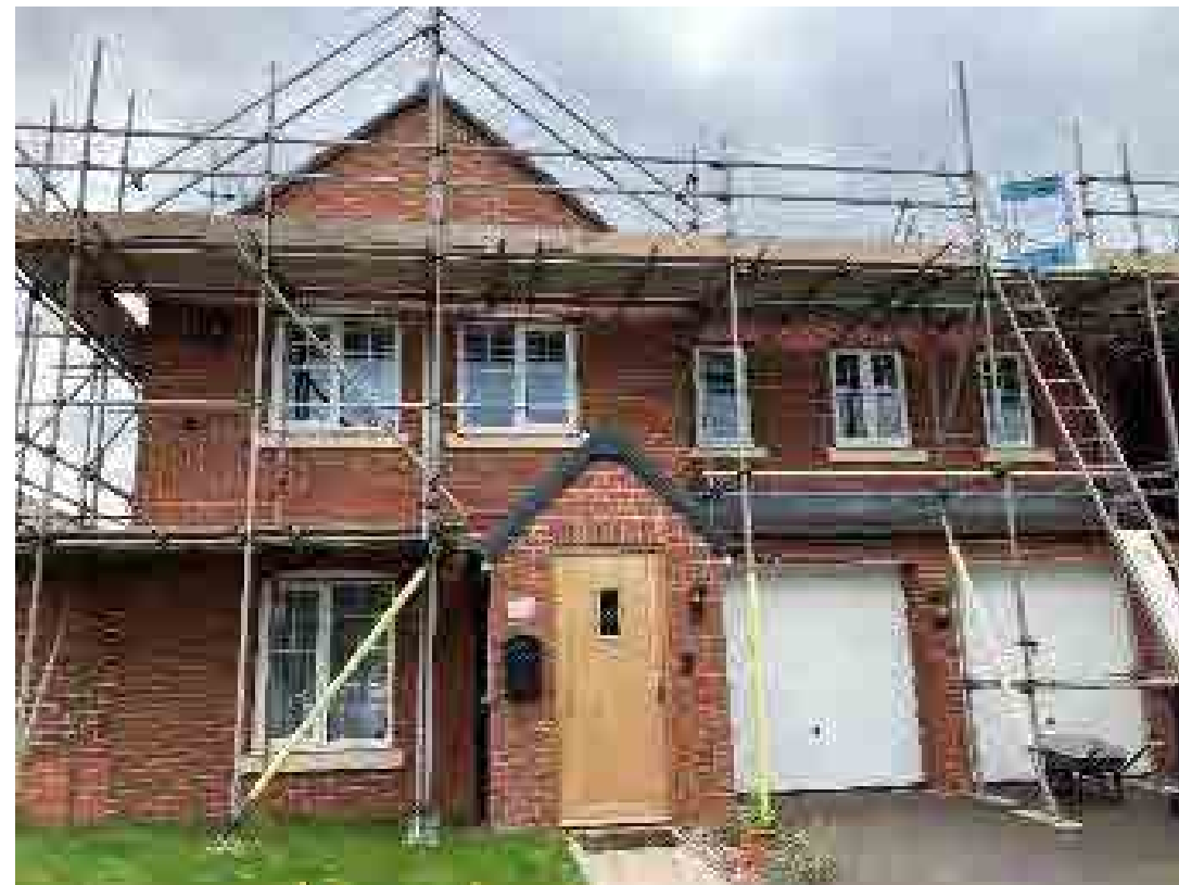
Full scaffold to gain safe access – significant inconvenience & cost
