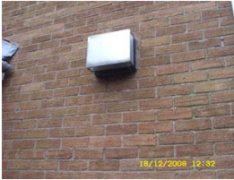
Balanced Flue
