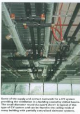
Simple constant volume air-conditioning system
