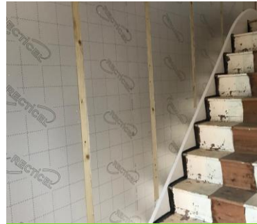
PUR/PIR Boards applied on a wall
